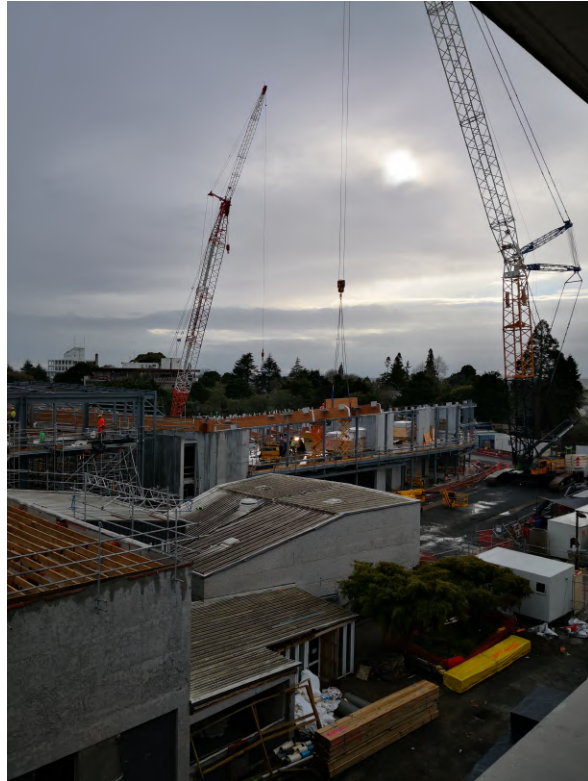
Figure 5: Pa/Student Centre construction August 2021
